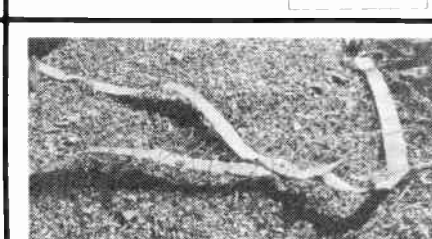
Photo 2. A poor ground system such as this one can cause unstable antenna resistance readings, making accurate power calculations difficult at best.
