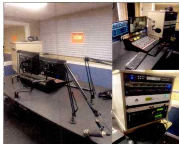
The Completed Studio
