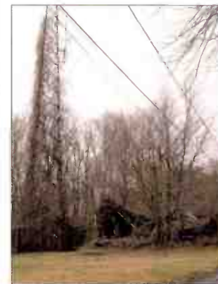
Abandoned 1960's vintage communication tower on site of former secret listening post.
