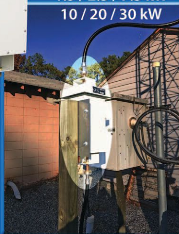
Kintronic supplied pre-fab tuning houses 1380 kHz WKDM - 1660 kHz WWRU Jersey City, NJ
