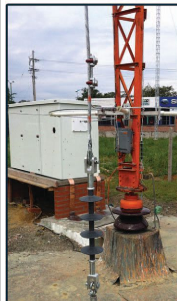
MODEL KSA-VCTB-10 KINSTAR LOW PROFILE ANTENNA ON THE AIR IN COLOMBIA, SOUTH AMERICA
