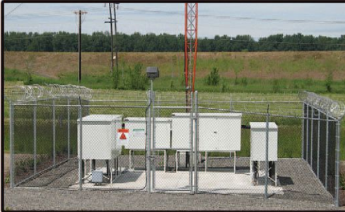
ENTERCOM DIPLEXED AM DIRECTIONAL ANTENNA SYSTEM, VANCOUVER-WA
