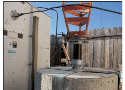
A new insulator supports the tower.
