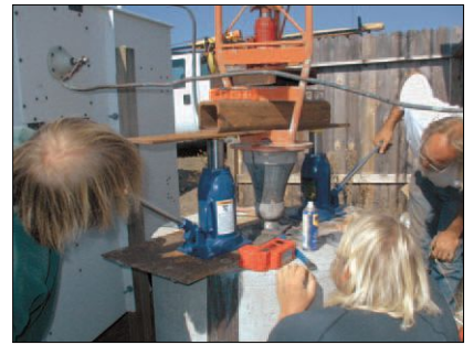
Slowly jacking the tower.
