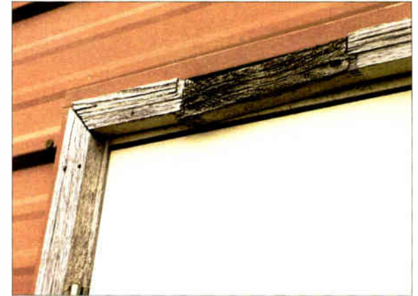
Poor maintenance by the previous owner. A door frame being destroyed due to neglect.
