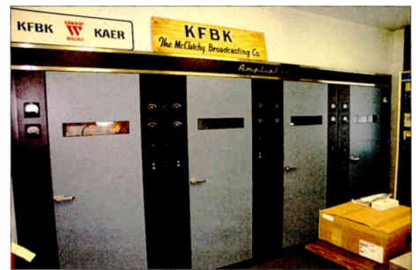
KFBK replaced its original 50 kW with this BTA-50H1S in 1969
