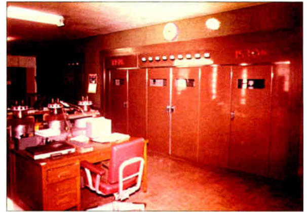
The McClatchey 50 kW transmitter. Notice the spare finals on the desk, base up. Courtesy: Dale Harry
