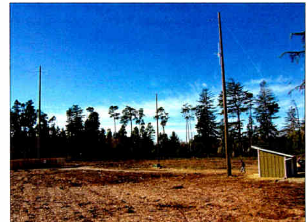
An overall view of the KCST Kinstar antenna, showing the center feed at the left, three of the five total support poles, and the transmitter building on the right. The STL dish is installed on the pole closest to the transmitter building.
