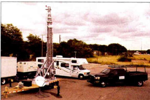
The ERT package includes a generator, a 100 foot tower (and obstruction light), a four-wheel drive pickup truck, and RV accommodations for staff.
