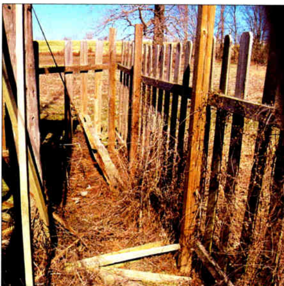
Fences not only protect the public from RF, they protect your copper from the public.
