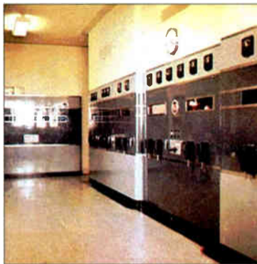
KTRH's 50-E and Phasing Cabinet Courtesy: Sam Lester
