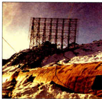
High in the Italian Alps (10,000 feet), Ken Branton helped install this antenna and two 831G-2C transmitters to pump RF into Zurich.
