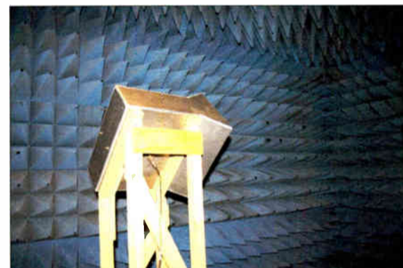
The indoor RF anechoic chamber.
