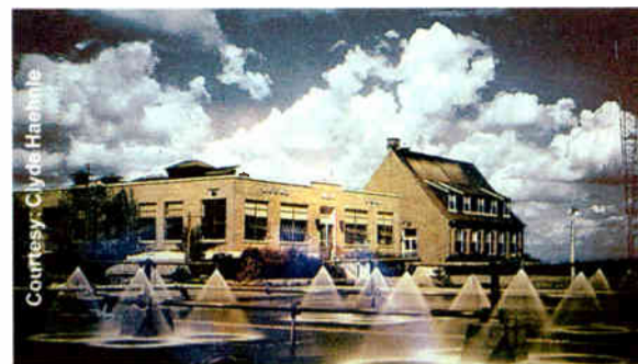
WLW's cooling pond was used to dissipate a lot of heat.
