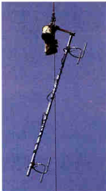
The antenna being hoisted to its mounting position.
