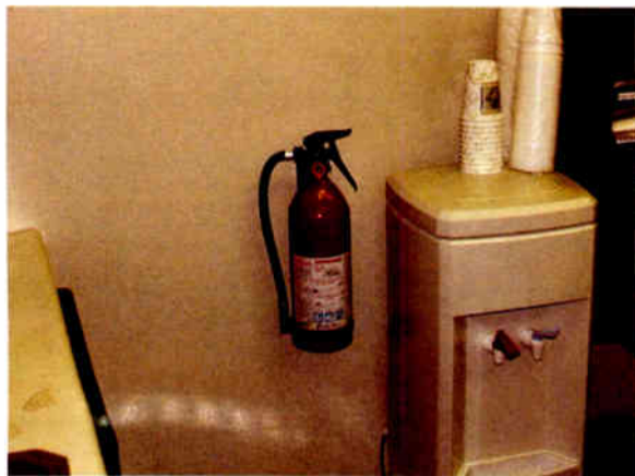
A fire extinguisher must be off the floor, but not so high as to make it hard to reach.
