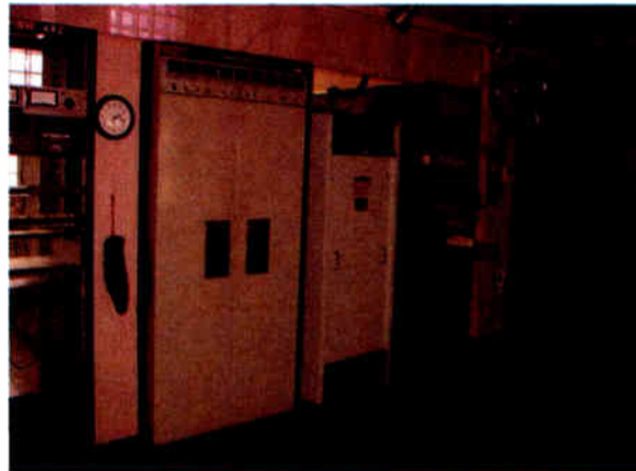
To help KQV "rock," ABC installed an ITA 5 kW transmitter.
