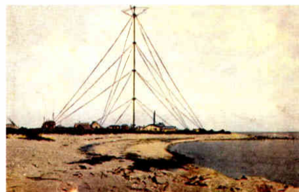
National Electric Signaling Company Brant Rock, Massachusetts
