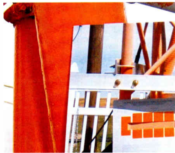
The properly repainted tower compared with the faded version.
