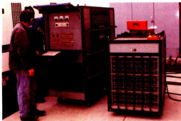
Using a load bank to fully test a generator.
