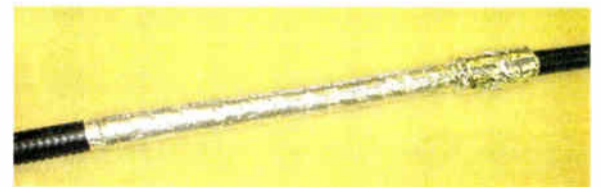
Closeup of Burnished Double Layer Protective Foil Upper Layers Overlap Lower Layers to Shed Moisture
