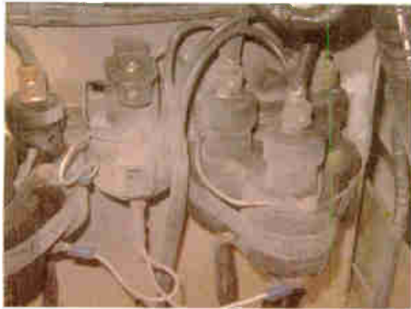
Exploded 3-phase plate transformer contactor using mercury switches.
