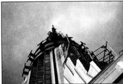
The 28-year old Alford antenna sits above the building's observation deck.
