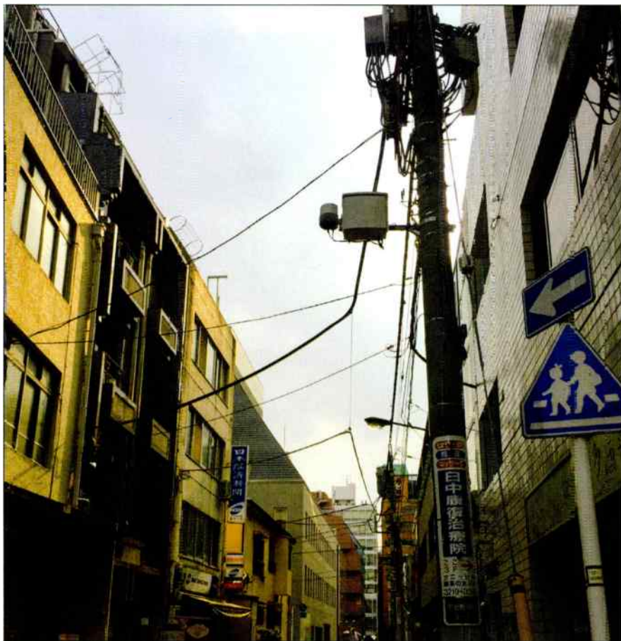
Photo 3. The node shown in the foreground is a typical street alley deployment. Its neighboring node is farther along the canyon.
