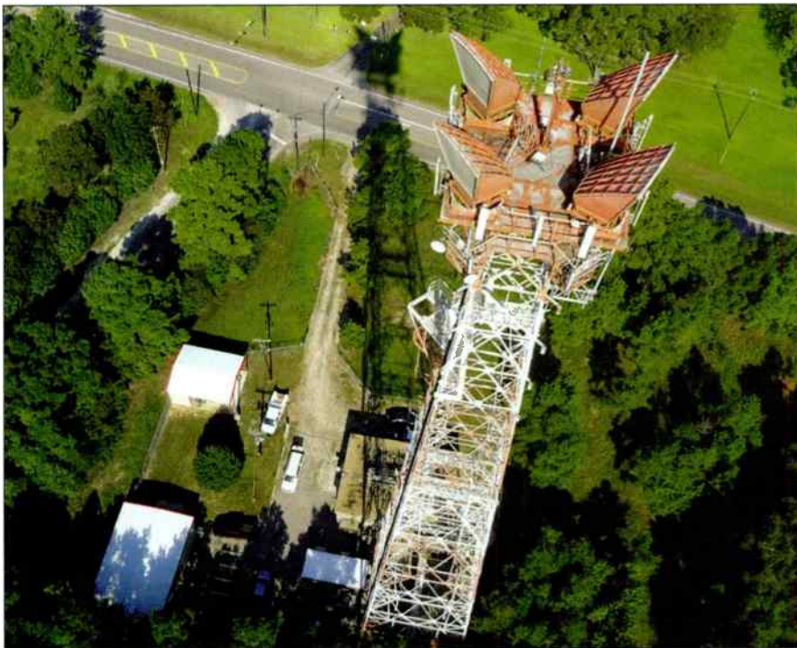
The author engaged the services of a UAS operator and a data analysis platform company to inspect his 263-foot tower in Willis, Texas. The horn antennas on top reveal the tower's origin as part of AT&T's Long Lines microwave network.
