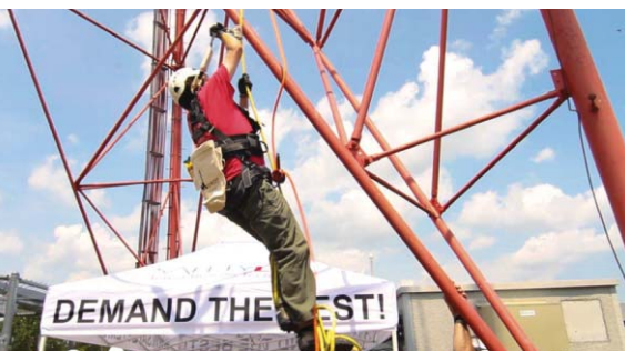
In the heat of the day, Biby can't quite muster the strength to lift the handle to unlock the fall-arrest mechanism. Jones directed him to maneuver over to the tower. Photos by Don Bishop
