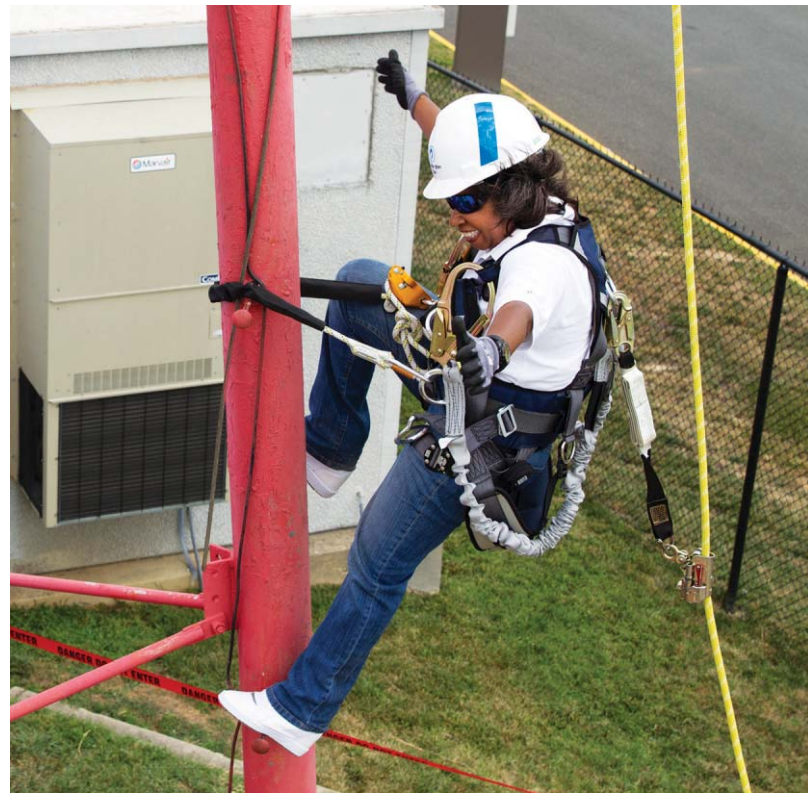
Thornton, vice president and general counsel, WGL Holdings and Washington Gas, completes a training exercise as she leans back in her safety harness and lets go of the tower. A lanyard connects the dorsal D-Ring on her harness with a locking mechanism on the yellow safety rope to provide fall-arrest protection. Photo by Don Bishop
