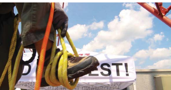
Biby makes three loops in his fall-arrest rope to anchor his foot. Then, he will push his body upward to reach for the rope lock.
