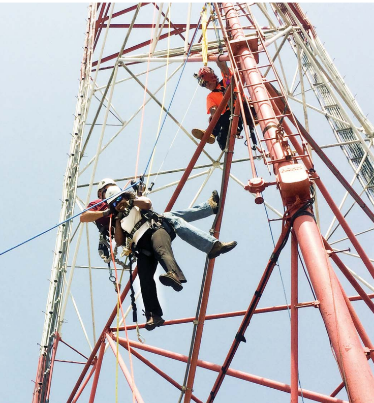
When the widely spaced pegs on the tower leg proved to be a climbing obstacle, crane operator Eric Severs used the personnel basket to lift Leslie T. Thornton to an elevation that allowed her to participate in a companion rescue exercise. Here, she plays the role of a victim who needs to be lowered from the tower to the ground. Photo by Binh "Alex" Nghe
