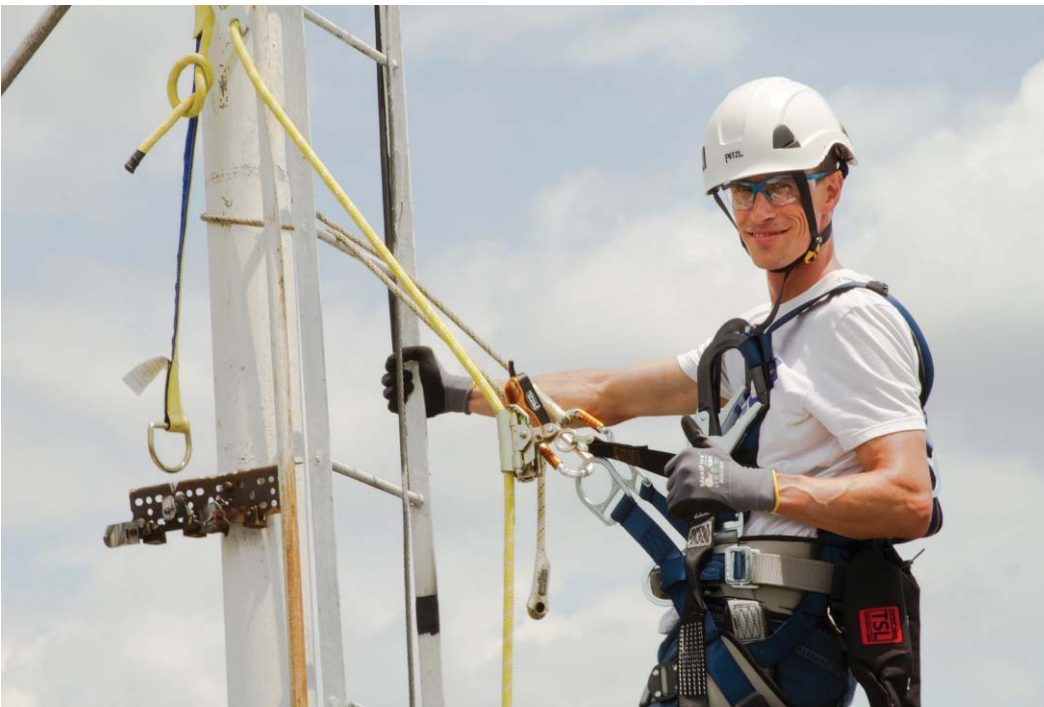
Eric Kampert, P.E., an occupational safety and health specialist for construction services in the OSHA Directorate of Construction at the U.S. Department of Labor, completed a training exercise by climbing to height while connected with a fall-arrest rope and placing another rope around the tower leg to secure his position. Photo by Don Bishop
