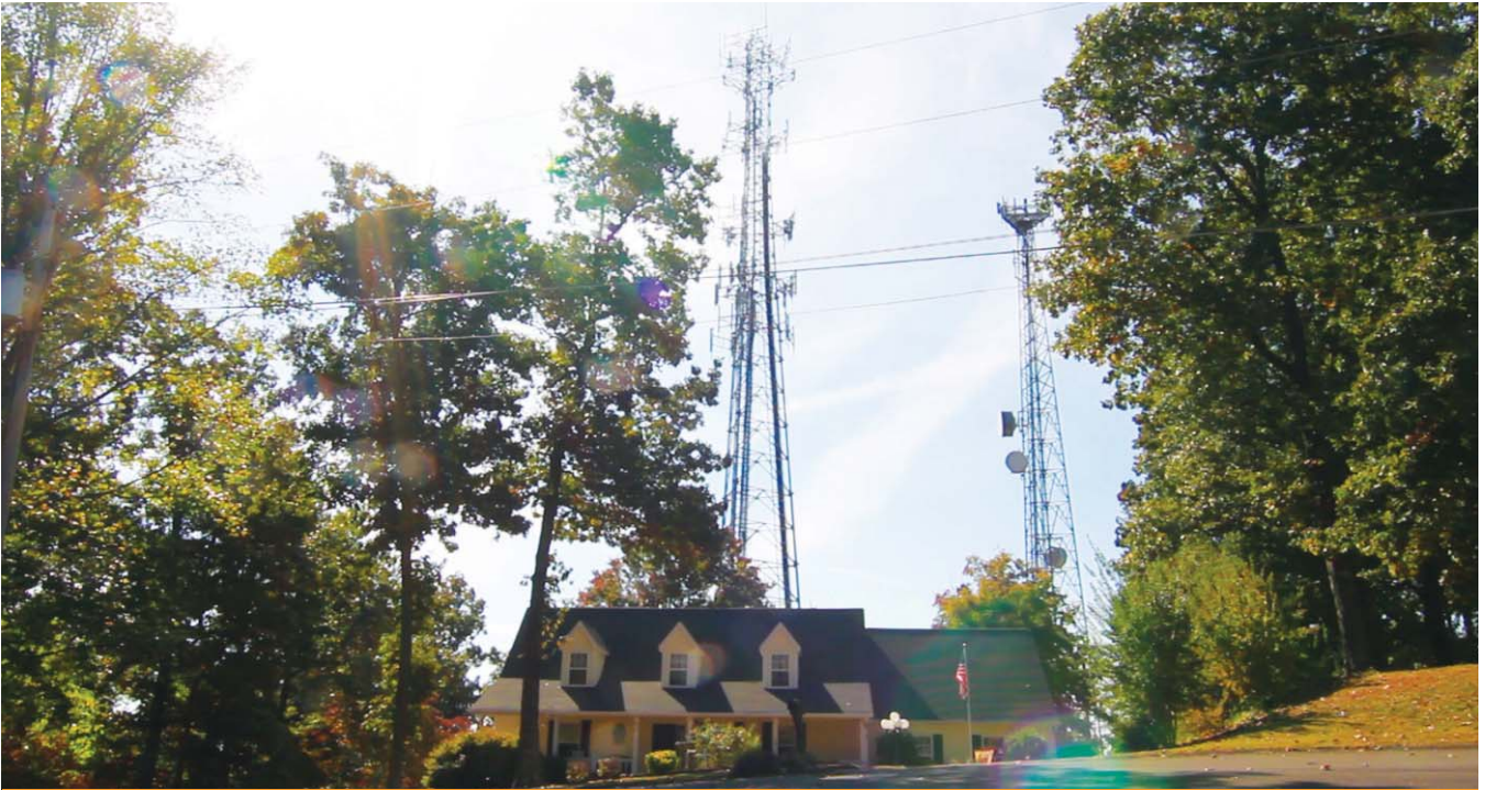
Wireless carriers use towers positioned behind a house in Cleveland, Tennessee. Photo by Don Bishop
