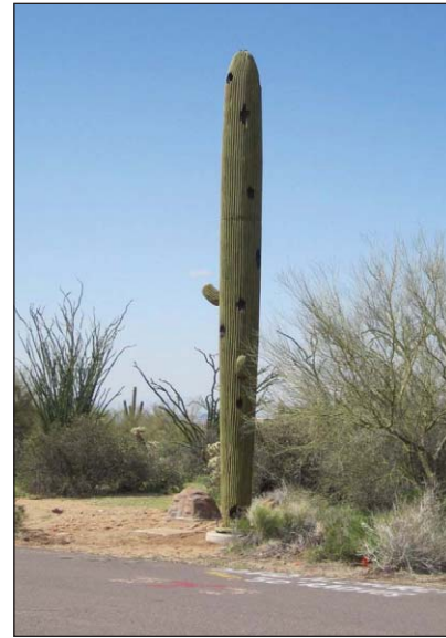
A faux cactus conceals a cellular base station and antenna.
