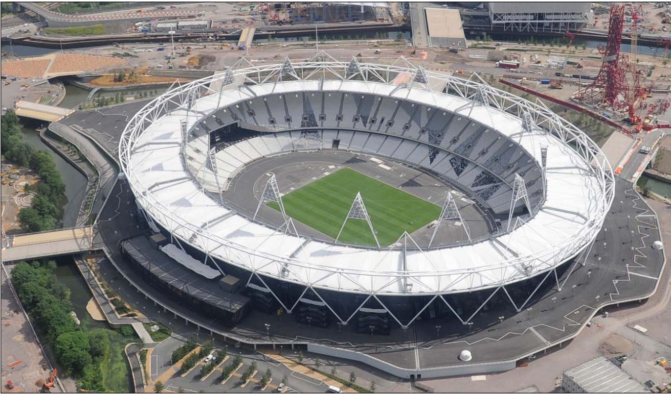
Photo 1. Positioned between two waterways on a diamond-shaped island, the London Olympic Stadium was equipped with a distributed antenna system capable of serving mobile wireless users among as many as 80,000 spectators attending events in the stadium.
