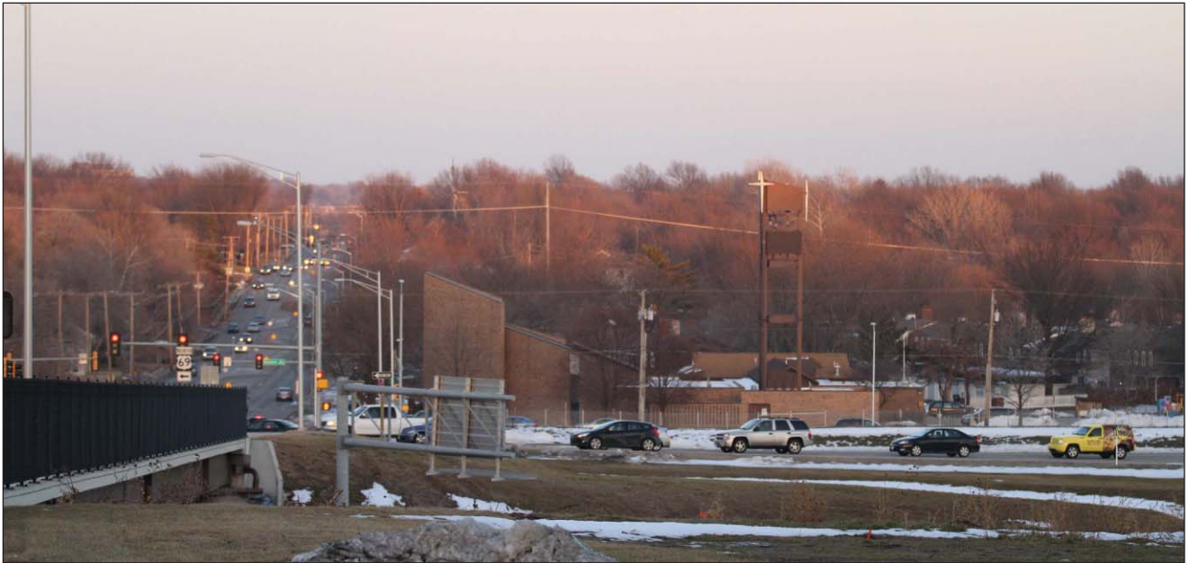
Where it stands at a church near a freeway, a cell tower with a cross at the top blends into the background. Several wireless communications carriers share the tower with their antennas concealed behind panels extended between the tower's legs.
