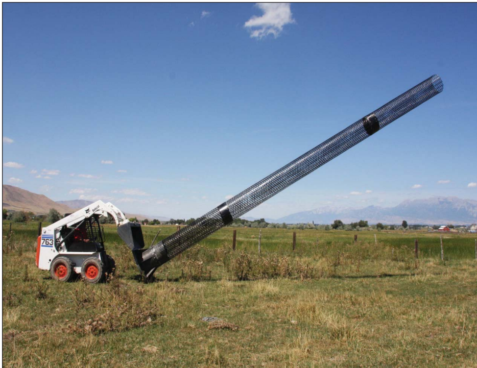
Photo 3. A carbon-fiber structure is so lightweight that a compact excavator is sufficient to move it about and stand it erect.
