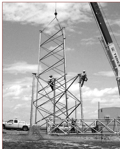
Photo 1. Tower technology has been stagnant for 20 years. Reducing cost means reducing capacity. For backup power, many sites rely on diesel generators. The capex and opex of passive infrastructure remain high.
