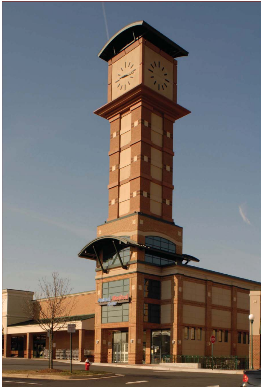
Photo 2. A site designed to look like a clock tower conceals antennas placed above a building's roofline. Load-bearing limitations of a building's infrastructure may limit how much wireless communications equipment can be placed inside such a concealment to less than what may be possible with freestanding structures.
