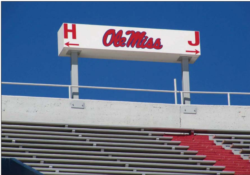
Photo 4. In stadiums, signage can be used to conceal antennas used as part of distributed antenna system (DAS) networks.
