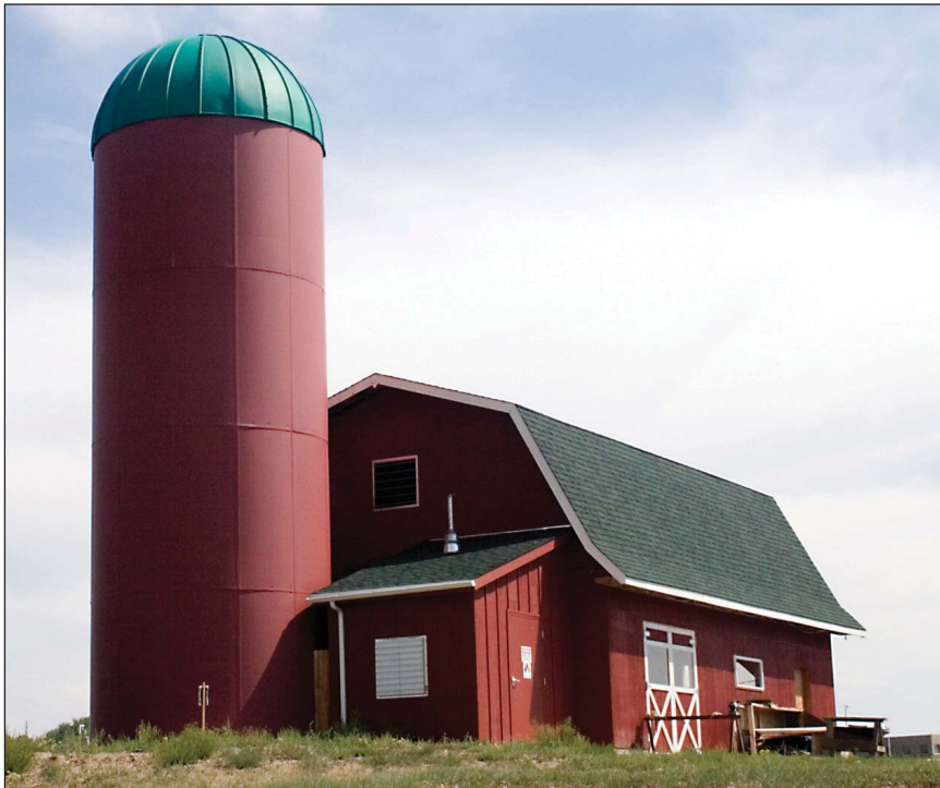
Photo 3. As a freestanding structure, a silo has the potential to be constructed with more load-bearing strength than a rooftop or the side of a building may have.
