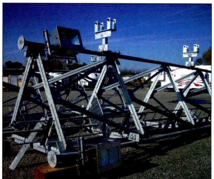
The third of four tower light levels is shown here already installed prior to being hoisted up. It is good to have an opportunity to inspect them while the tower is on the ground, which is the last time non-climbers can photograph the flash heads.
