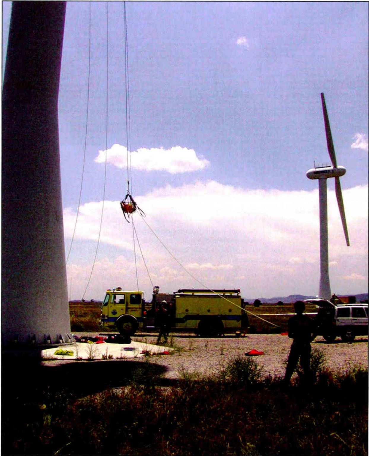
The scene above shows rigging for a rescue training session using a U.S. Department of Energy wind turbine. The rigging is used to conduct simulated rescues from the platform 128 feet high on the turbine. Safety One's Steve Fleming conducted the training for the Cherryvale Fire Protection District located south of Boulder, Colo. The district is under contract with DOE to provide rescue service at the site.
