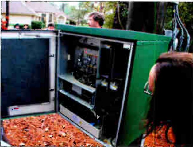
A visitor looks inside the equipment box at the base of a DAS node in Hilton Head Island, SC, during a tour arranged by the DAS Forum.
