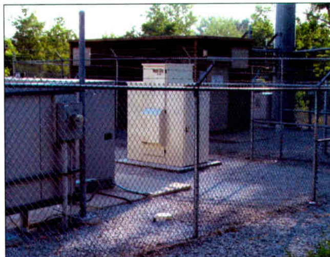
Fuel-cell systems require a relatively small footprint at a tower site, and their lack of combustion noise enhances their appeal for sites near residential or mixed-use neighborhoods.
