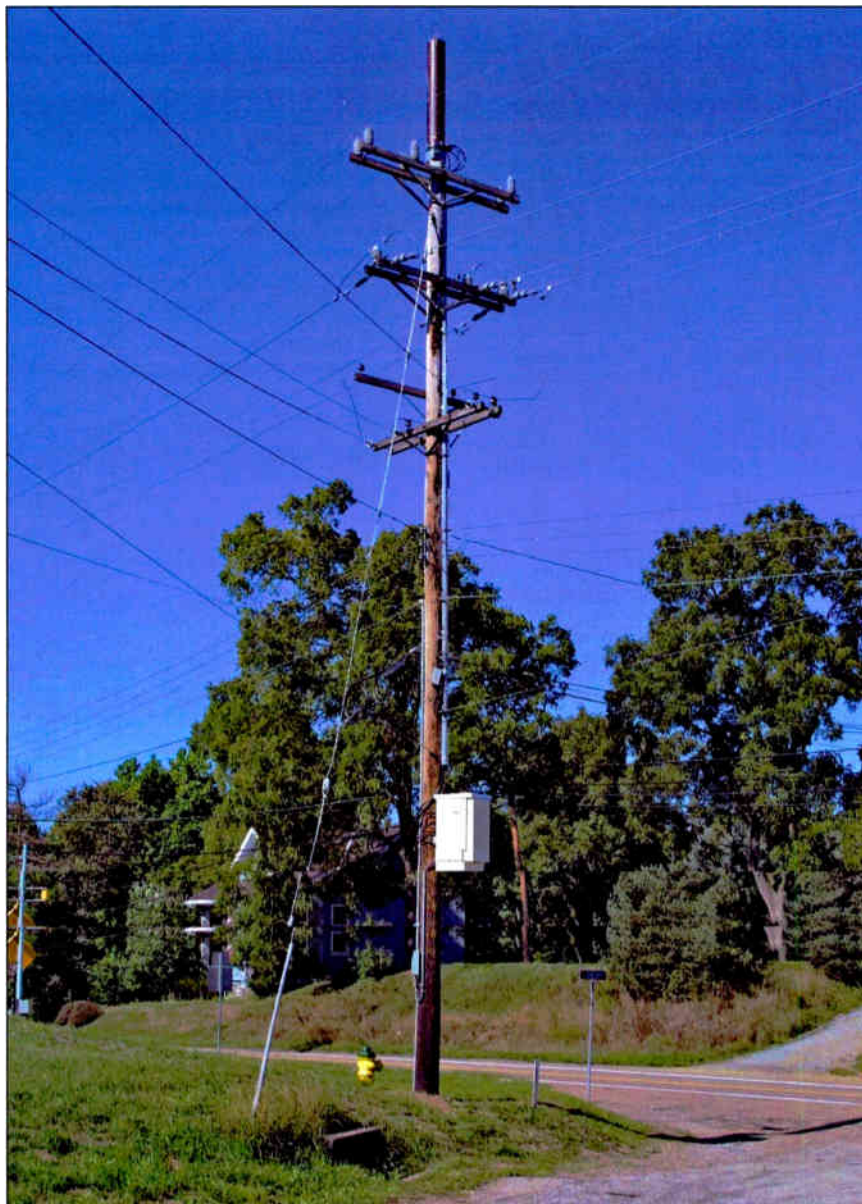
A utility pole may already be crowded with cross arms and wires that probably weren't subject to zoning. The addition of an antenna should not raise zoning issues. In this picture, the antenna is top-mounted in a radome. Photo courtesy of ADC Telecommunications and Phazar Antenna Corporation
