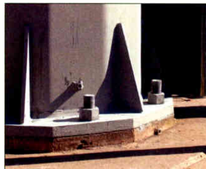
Base plate with stiffeners.
