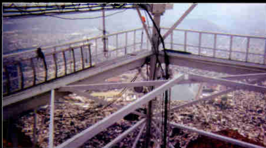
Some tower structures have rings or platforms, but generally there is no flat area for worker rest or equipment assembly. Photo courtesy of ComTrain.
