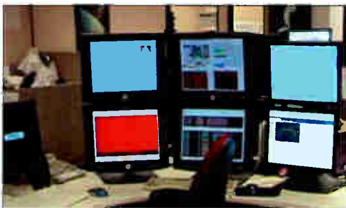
Linux-based systems enable low-cost ‘real estate’ for monitoring network operations.
