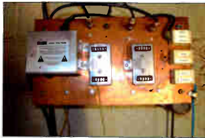
A finished common-ground mounting plate inside an equipment shelter.
