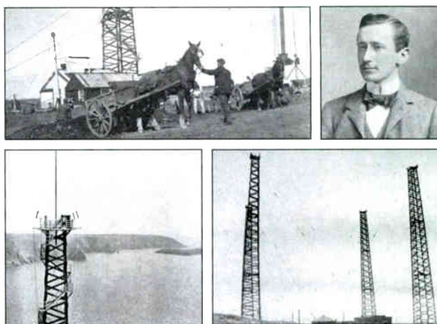
Clockwise from top left: (1) Reconstruction of towers at Poldhu, Cornwall, England, circa 1912; (2) Guglielmo Marconi, circa 1901; (3) Aerial towers at South Wellfleet, Cape Cod, MA, circa 1902; (4) View across Mullon Cove, Cornish Coast, from the top of another of the towers at Poldhu Station, circa 1901. Source: Marconi plc
