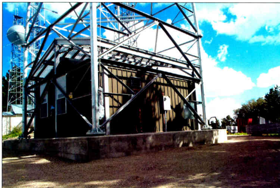
Site management encompasses all activities and property associated with the tower and equipment. Photo by Sabre Communications
