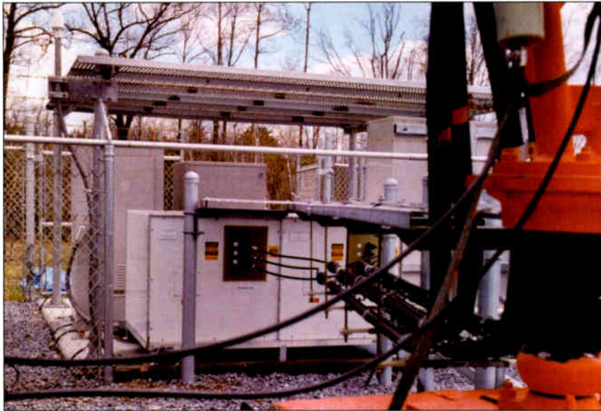
The CoLoCoil system isolates multiple wireless coaxial cables with a modular approach that also allows adding more wireless carriers to the system.
