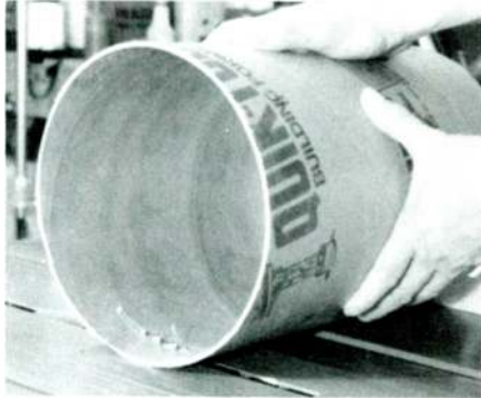
PHOTO 1: Cutting the tube to length.
