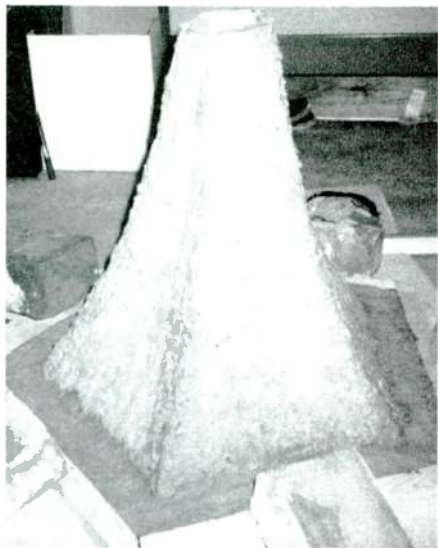
PHOTO 8: Casting the flange.
