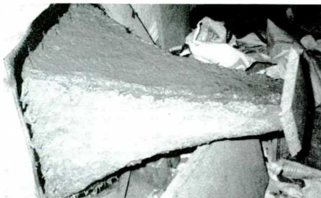
PHOTO 6: Applying concrete to speaker side. (Speaker is positioned sideways.)
