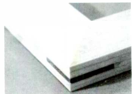
PHOTO 10: Complete spline corner joint.
