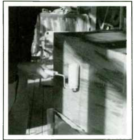
PHOTO 5: Roller coating with epoxy.
