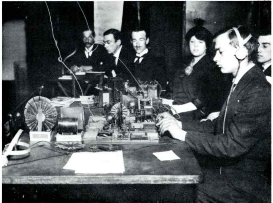
Fig. 1. The young Paul Voigt (with earphones) demonstrates a reflex (dual high and low frequency) amplifier circuit for the Wireless and Experimental Association of Peckham in 1922.
