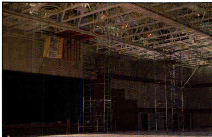
Ancha's Activity Center install-in-progress at Willow Creek.
