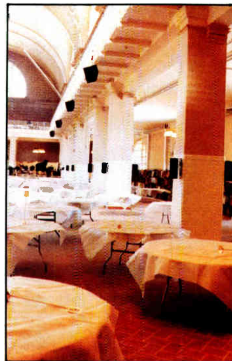
Meyer UPM-1As on columns; Meyer UM-1As hung from balcony. Note cables are hidden.
