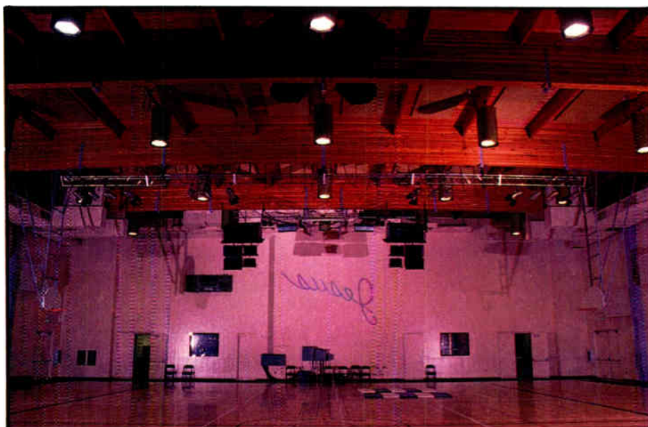
Front stage wall is lightly treated with Armstrong acoustical tile to minimize reflections from stage monitors.
