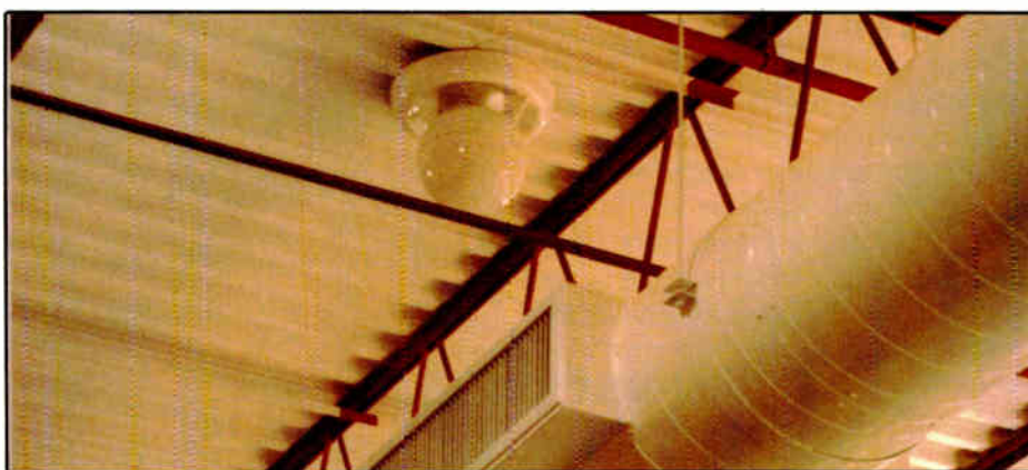
Three Soundsphere 110/A speakers were suspended from the ceiling for simplicity.
