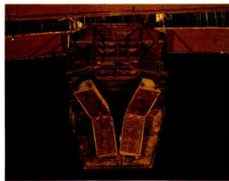
One of 10 clusters in the showroom using JBL Professional Concert Series components. This cluster is rigged to fly in and out of position for service.
