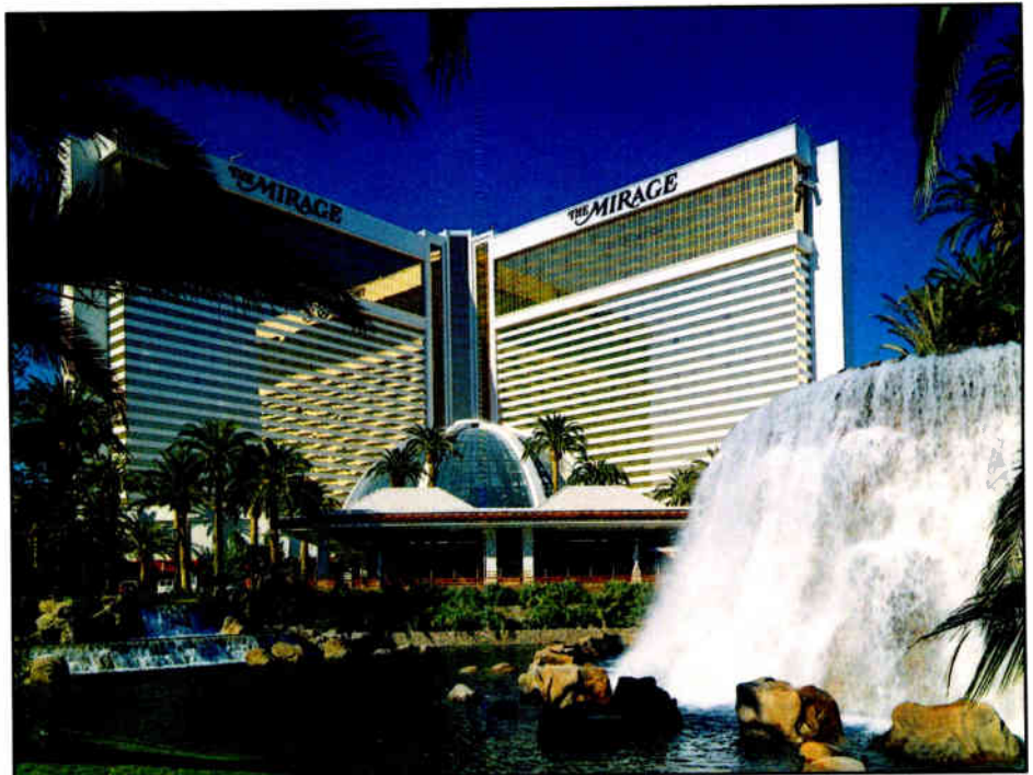
Stephen Wynn's Mirage Hotel is one of the world's largest. It was a model of fast track design-build construction.
