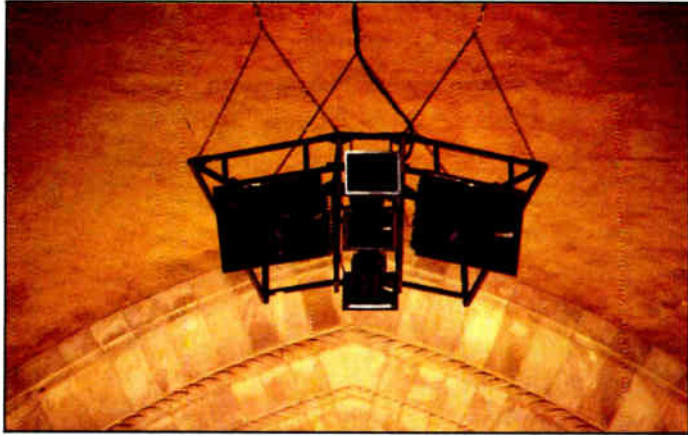
The central cluster: three Community horns, two M-80s (with 12-inch JBLs).
