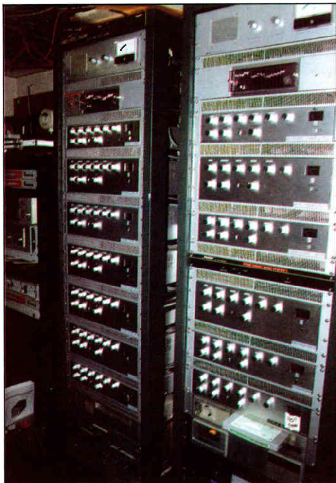
Equipment rack at the Sands.
