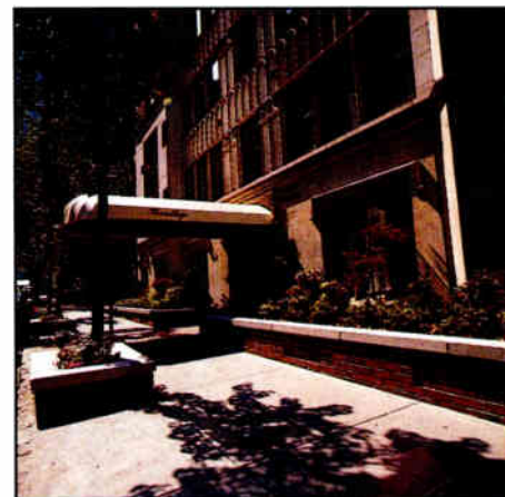
The Hermitage: Renovations offer opportunities for system upgrade.
