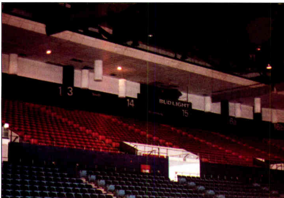
A few of the 100 Helmholtz radiators installed around the arena.
