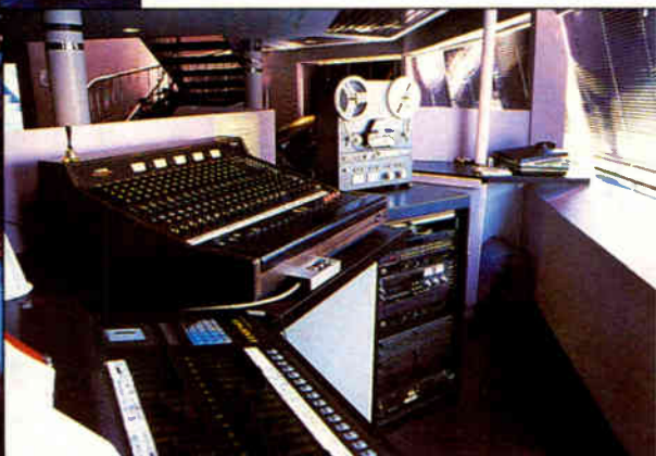
Lindy's Cabaret equipment set-up is similar to the Ballroom's. It includes a Yamaha 916 console, Tascam 122 cassette, Tascam 22 reel, Yamaha SPX 90 reverb, and Delta Lab CE 1700 DDL.
