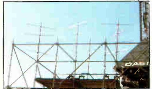
Yagi transmit/receive antennas near control pyramid.
