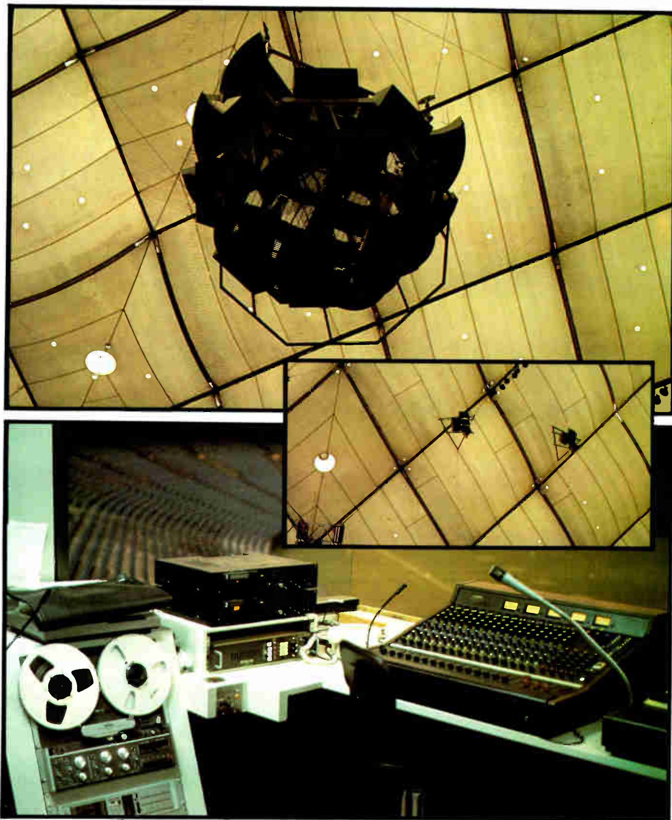
(Top) A view of the main loudspeaker cluster from below. Two satellite clusters (inset) are suspended on cables from the stadium's teflon-coated fiberglass roof. The soundbooth (bottom) at B.C. Place overlooks the entire stadium.
