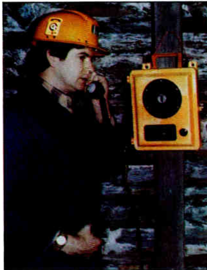
GAI-Tronics mine page in use in an underground coal mine.
