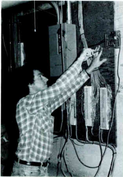
Installing the single-line autodialer.
