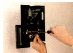
Step 3: Terminate wiring and position docking plate.
